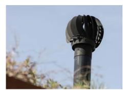
If there is a need to make curves to the ventilation line, we recommend adding a wind fan to increase air suction and evaporation.
